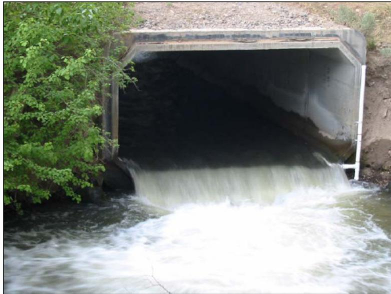
Figure A-1. Culvert 1 outlet. Note the stage recorder installed in the stilling basin on the right-hand side of the photo. The PIT tag antenna was not installed at the time the photo was taken.
