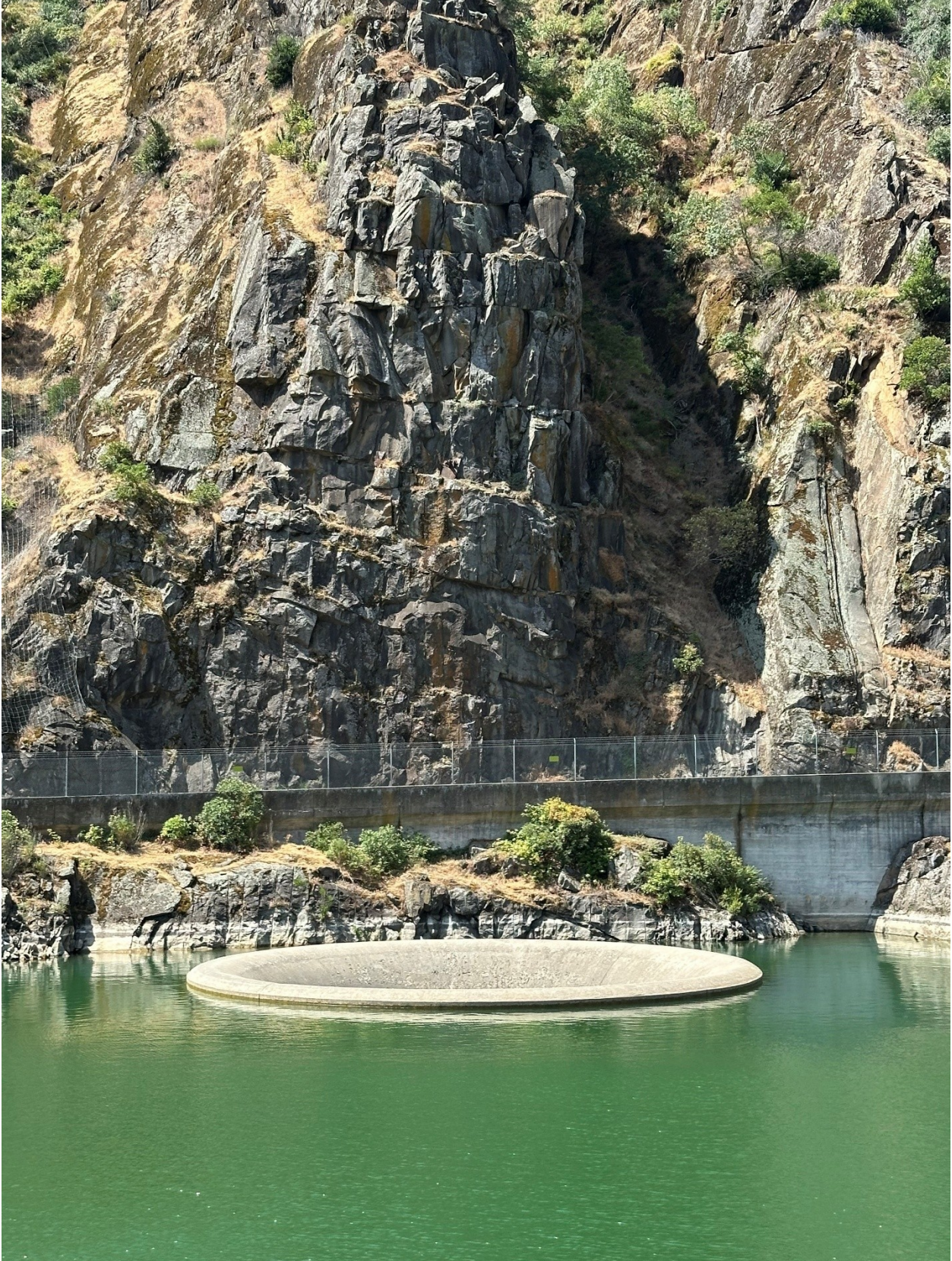
Figure 6-2. Lake Berryessa spillway (photo taken June 4, 2025).
