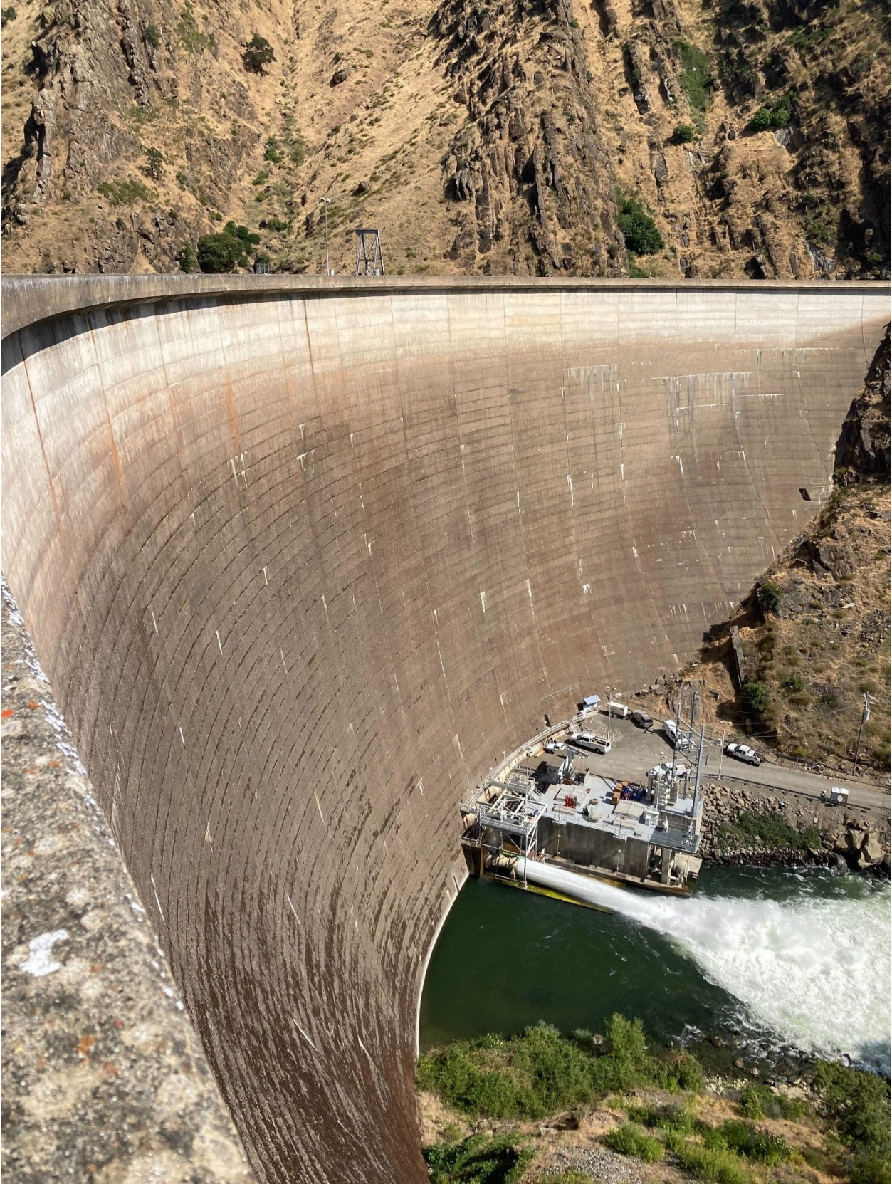
Figure 6-1. Face of Monticello Dam and outflow (photo taken June 4, 2025).
