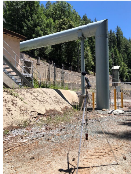
ST-1 Looking Southeast
