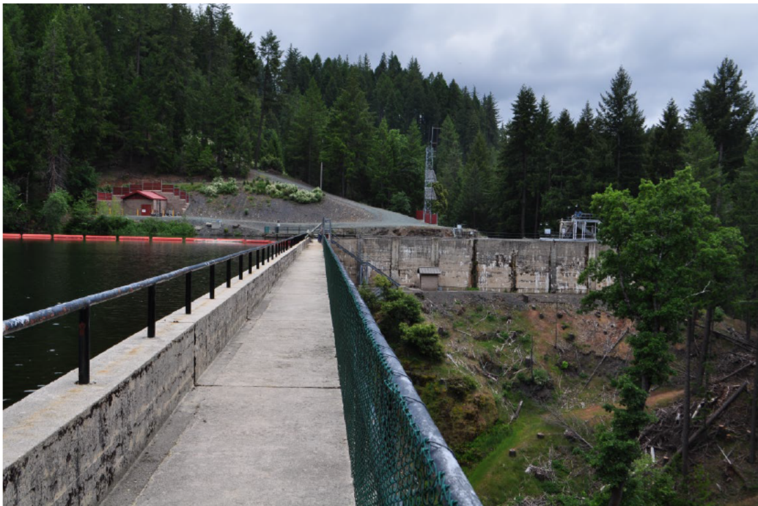
Key View 6. View from the dam walkway looking southeast toward the electrical control building, radio tower, and existing spillway structure.
