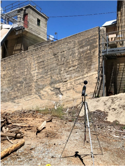
ST-1 Looking North
