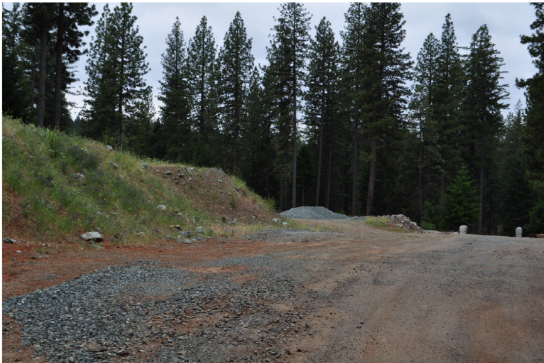
Key View 2. View looking southwest toward the existing staging and proposed spoils disposal area located off Salt Springs Road.
