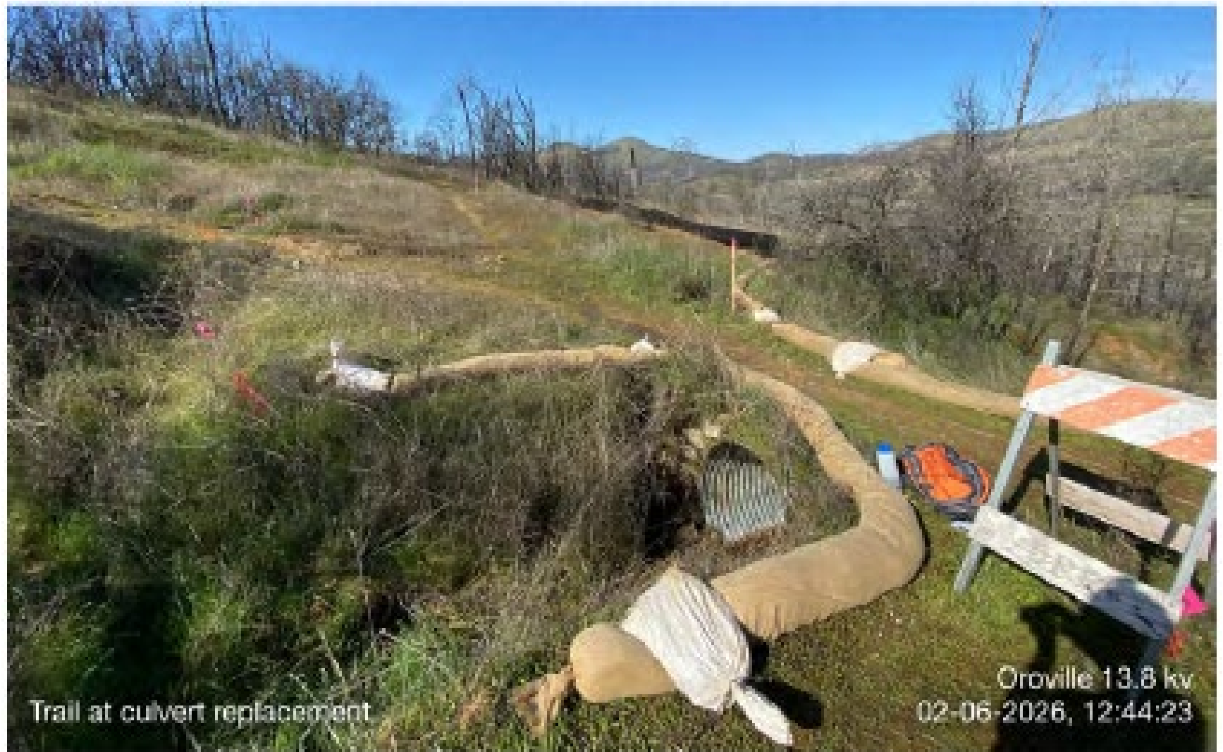
Figure 2: Oroville 13.8kV Transmission Line and Fiber Optic Replacement Project Culvert Replacement
