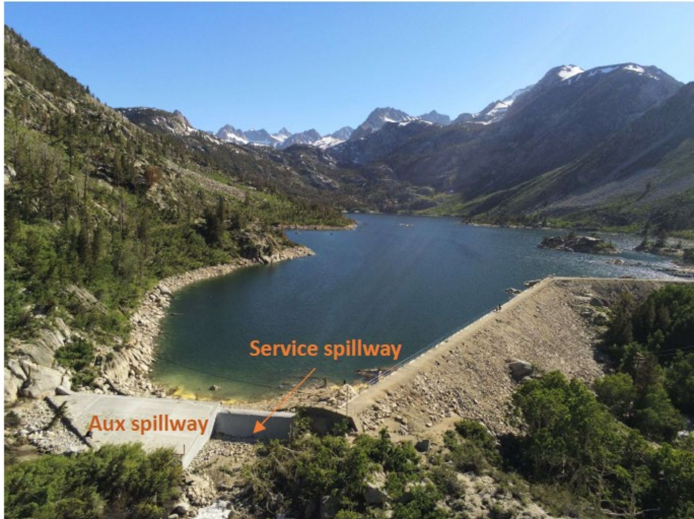
Figure 3: Existing Sabrina Spillway
