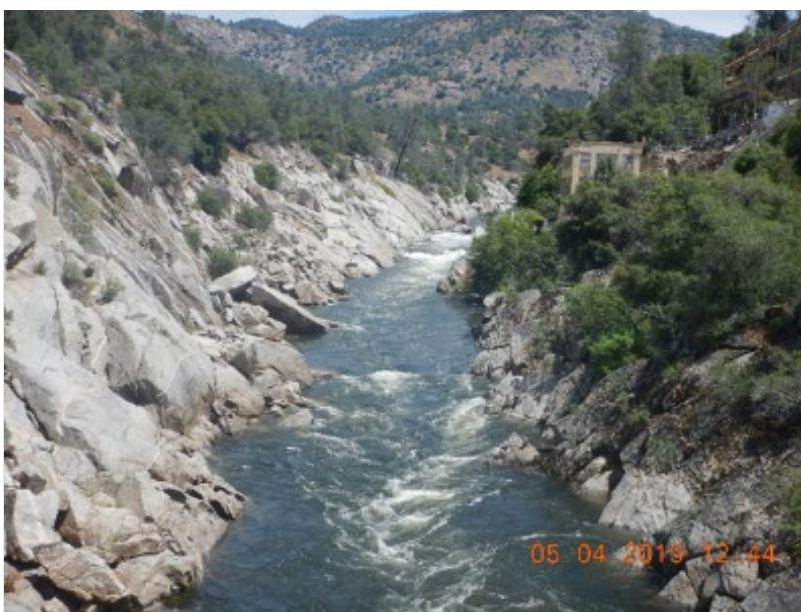
Figure 4.1-3: Key Viewing Area 3 – United States Bureau of Land Management Footbridge Crossing the San Joaquin River Downstream of the Kerckhoff 1 Powerhouse
